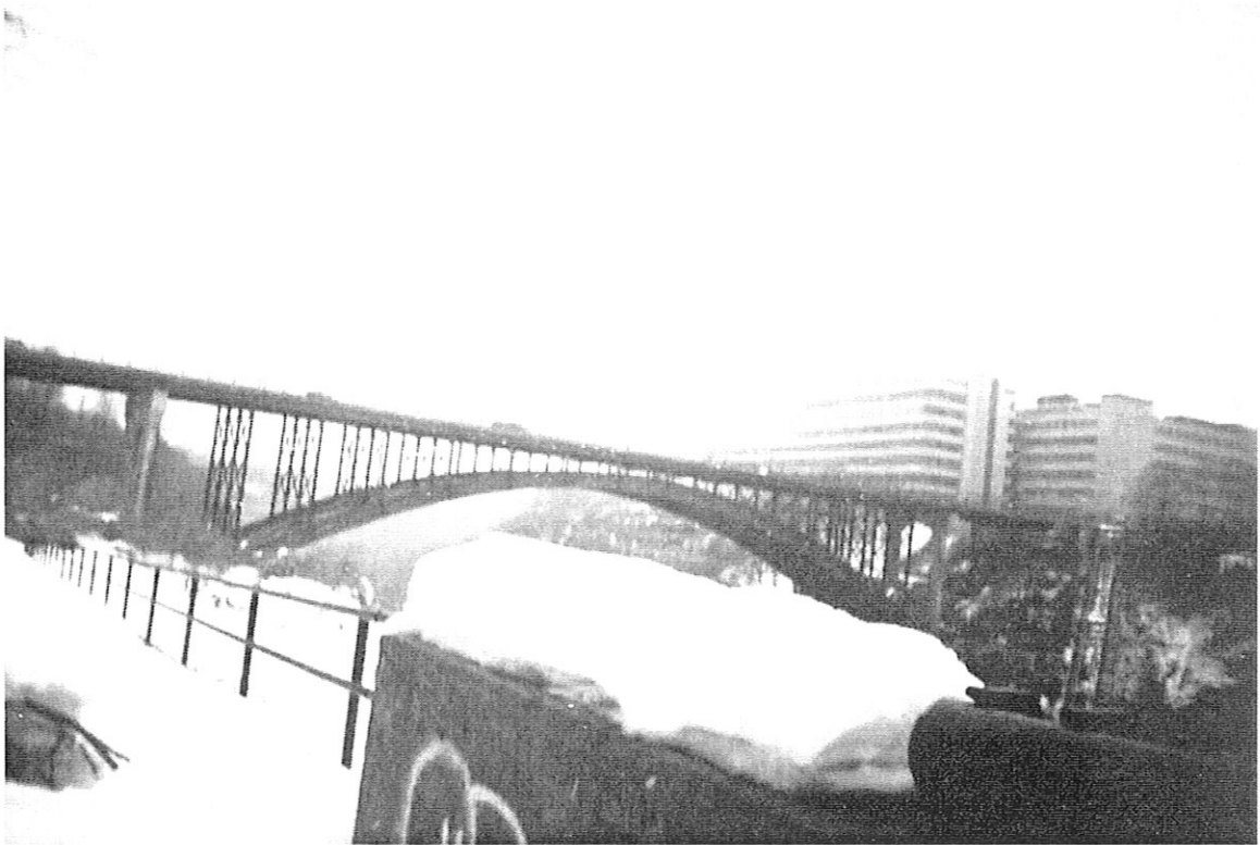
This is the Driving Park Bridge. It was winter when we went. This is an arch bridge in Rochester.
