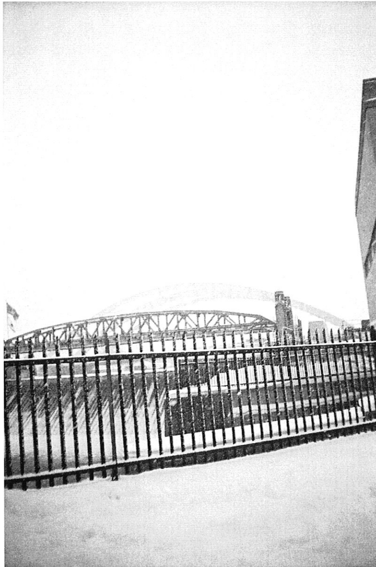
This is the Troup-Howell Bridge. It is a new bridge. It makes it easier to cross the Genesee River. It is in downtown Rochester. I cross it every time I go to my Grandma's house.
