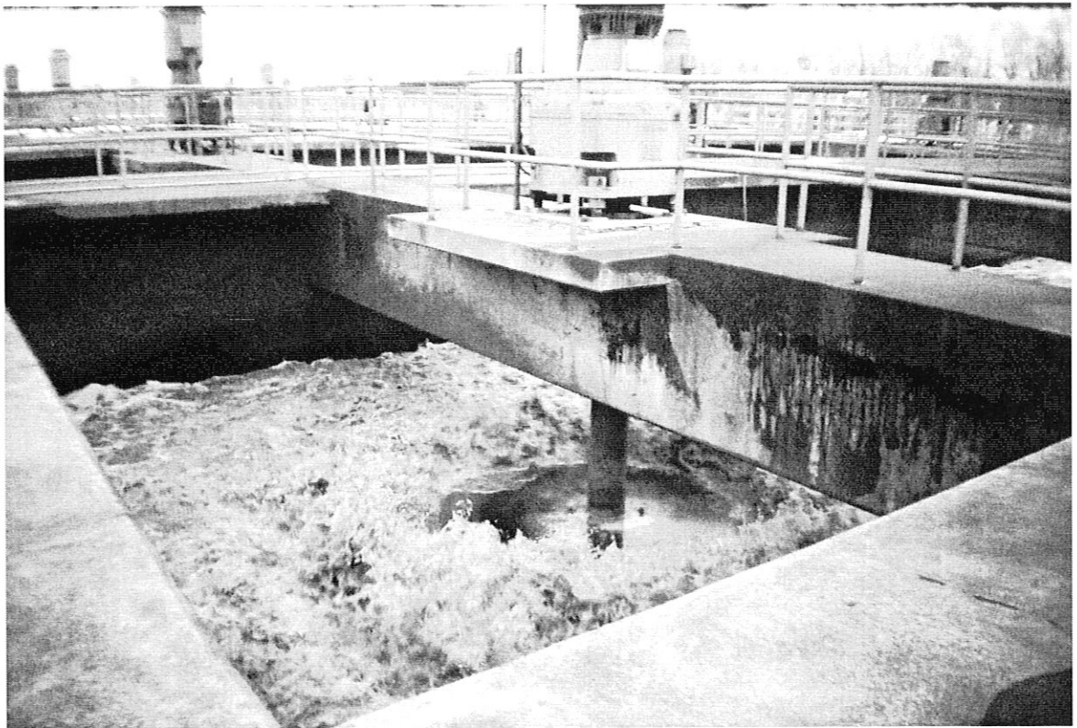
This is the aeration basin at the Sewage Treatment Plant. It was taken in February 2007.
