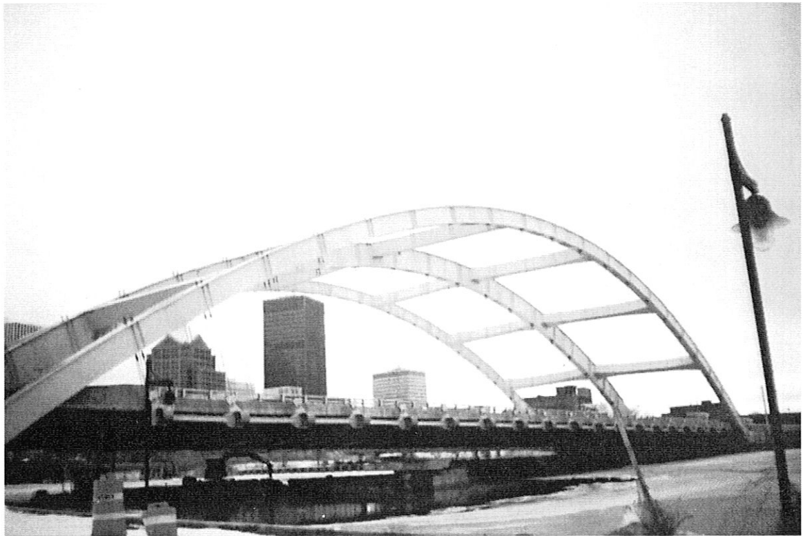
This is the Troup-Howell Bridge in Rochester. It is safe to go over. I took the picture in the winter of 2007.
