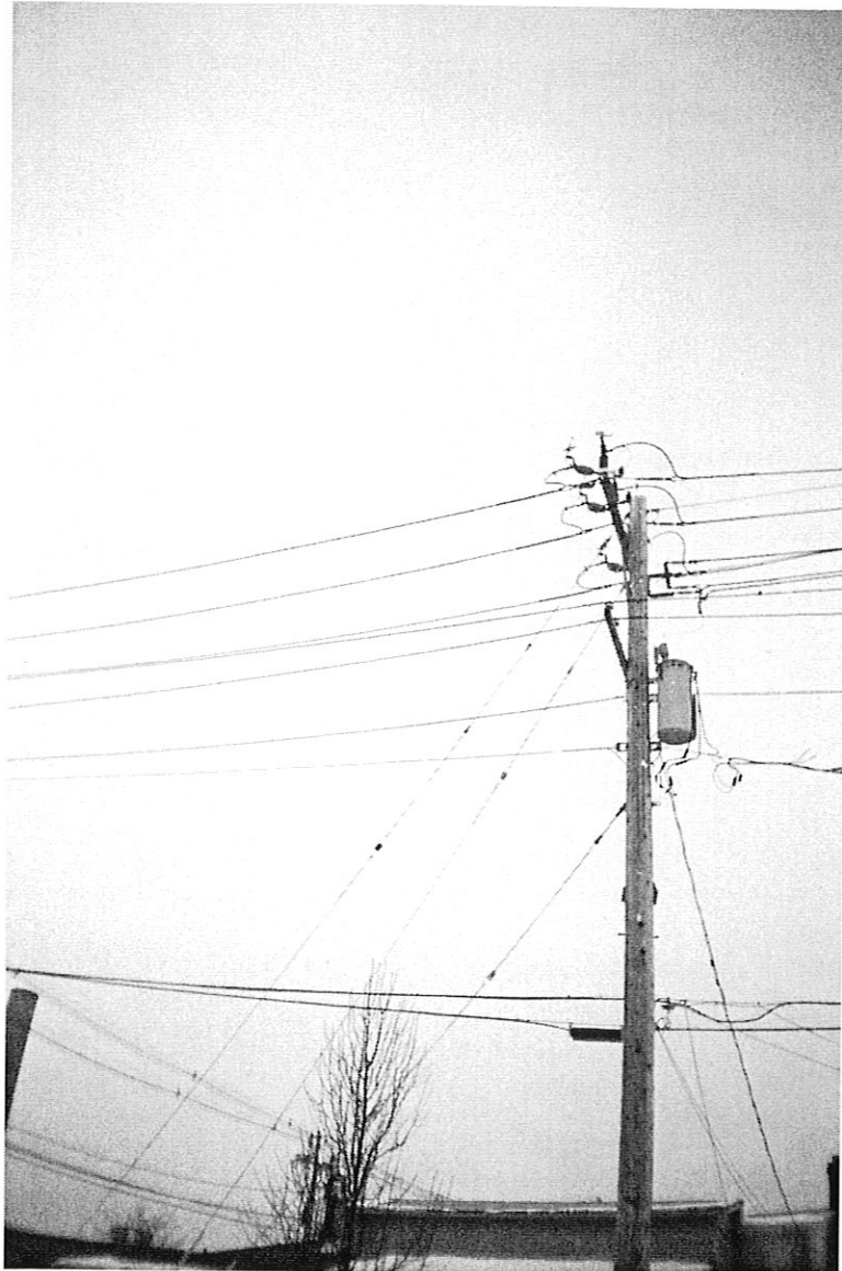
This is a transformer! It lowers electricity. This was taken at Faiport Electric on Monday, February 12, 2007.
